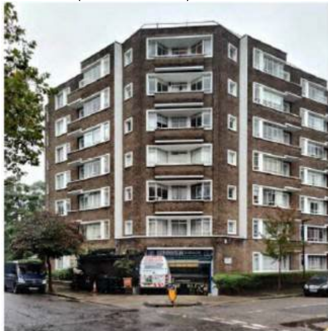
View of northern elevation at the junction with Newcourt Street and Culworth Street
